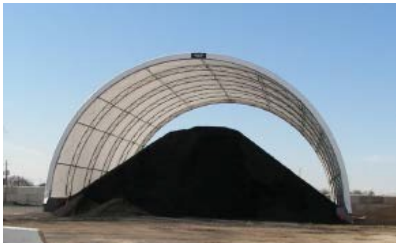
FIGURE 8 RAS Stockpile Covering (23)
