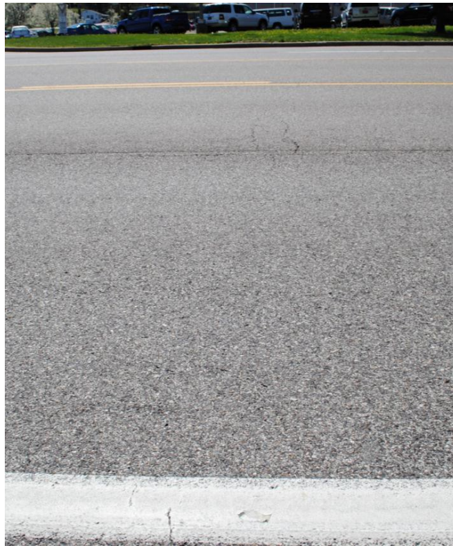
FIGURE 3 MoDOT RAS Pilot Project after Six Years (18)
